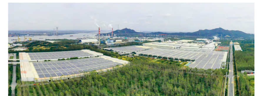
Phase III of Gold East Paper's 20-MW rooftop photovoltaic project
